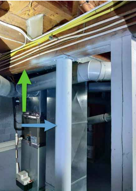
Main Beam (Green) and Support Column (Blue)
