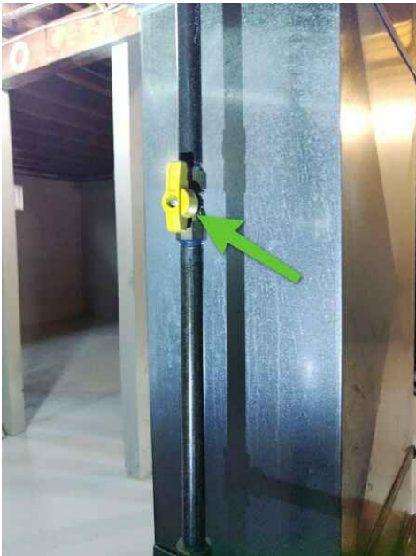
Gas Shut Off Valve
