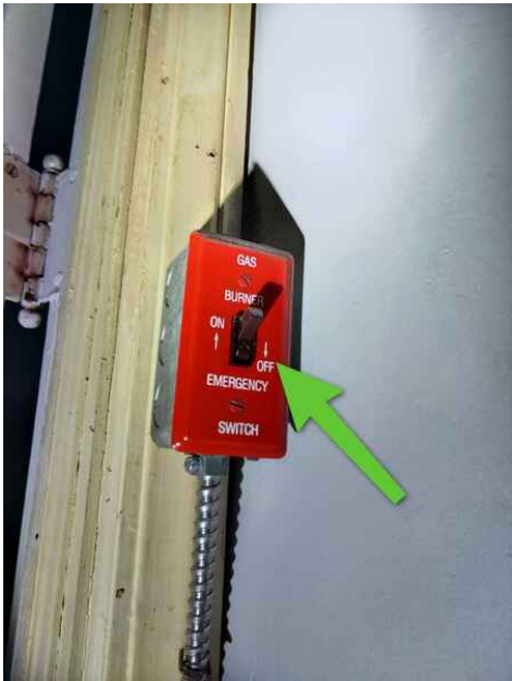
Emergency Shut Off Switch - Stairway
