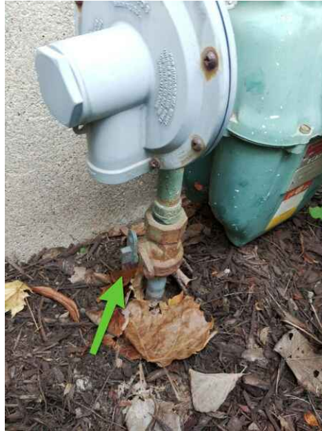
Main Gas Shut Off Valve
