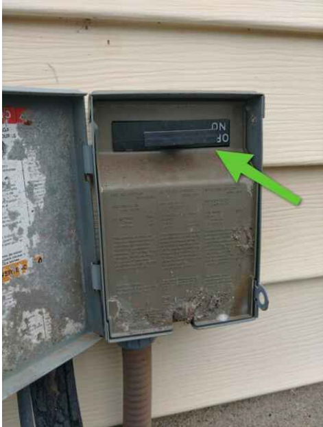
Main Electric Disconnect
