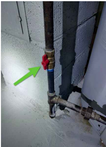
Gas Shut Off Valve
